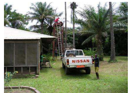
Pete Doerksen and Everett Halstead install a water tank in Tarencha.
